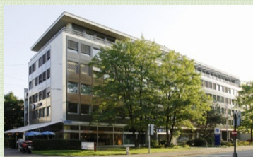
Basel, St. Alban-Anlage 46 rentable area: 3'818 m 2
