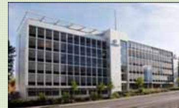
Bern, Eigerstrasse 2 rentable area: 4'676 m 2
