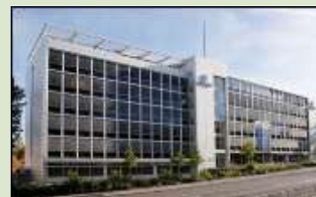
Bern, Eigerstrasse 2 rentable area: 4'676 m 2
