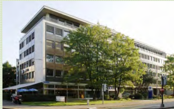
Basel, St. Alban-Anlage 46 rentable area: 3'816 m 2
