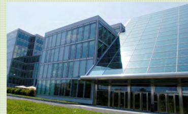
Lancy, Avenue des Morgines 8-10 rentable area: 15'855 m 2
