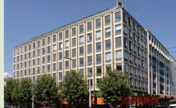
Geneva, Cours de Rive 13, 15 rentable area: 5'665 m 2
