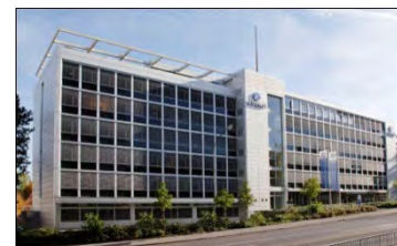
Bern, Eigerstrasse 2 rentable area: 4'676 m 2
