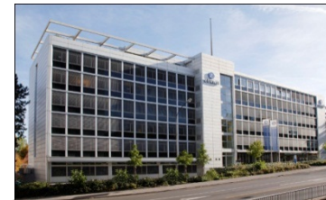
Bern, Eigerstrasse 2 rentable area: 4'676 m 2
