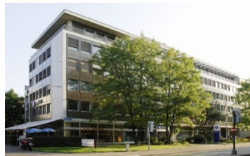
Basel, St. Alban-Anlage 46 rentable area: 3'816 m 2
