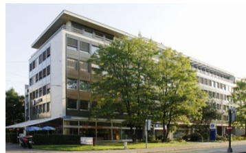
Basel, St. Alban-Anlage 46 rentable area: 3'816 m 2
