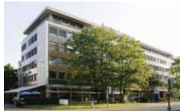
Basel, St. Alban-Anlage 46 rentable area: 3'816 m 2
