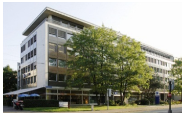
Basel, St. Alban-Anlage 46 rentable area: 3'816 m 2
