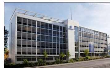
Bern, Eigerstrasse 2 rentable area: 4'685 m 2
