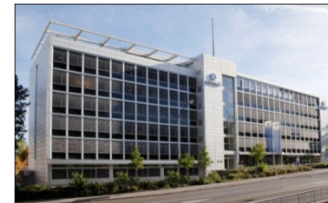
Bern, Eigerstrasse 2 rentable area: 4'685 m 2
