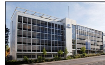
Bern, Eigerstrasse 2 rentable area: 4'685 m 2
