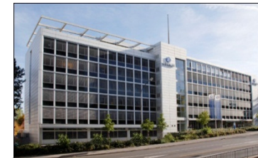
Bern, Eigerstrasse 2 rentable area: 4'685 m 2
