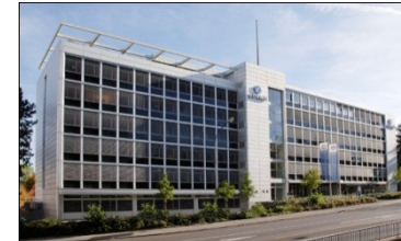
Bern, Eigerstrasse 2 rentable area: 4'687 m 2
