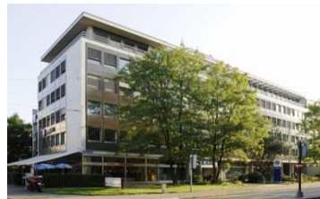
Basel, St. Alban-Anlage 46 rentable area: 3'805 m 2
