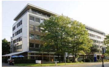
Basel, St. Alban-Anlage 46 rentable area: 3'773 m 2
